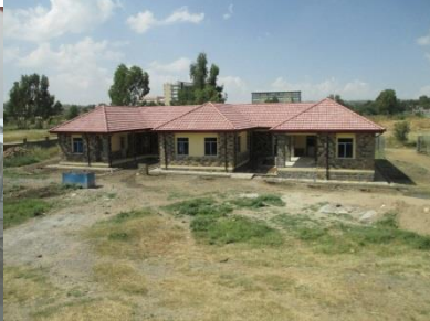
High school staff building
