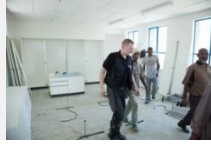
Assembling the furniture
