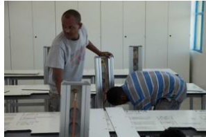
Assembling the utilities posts
